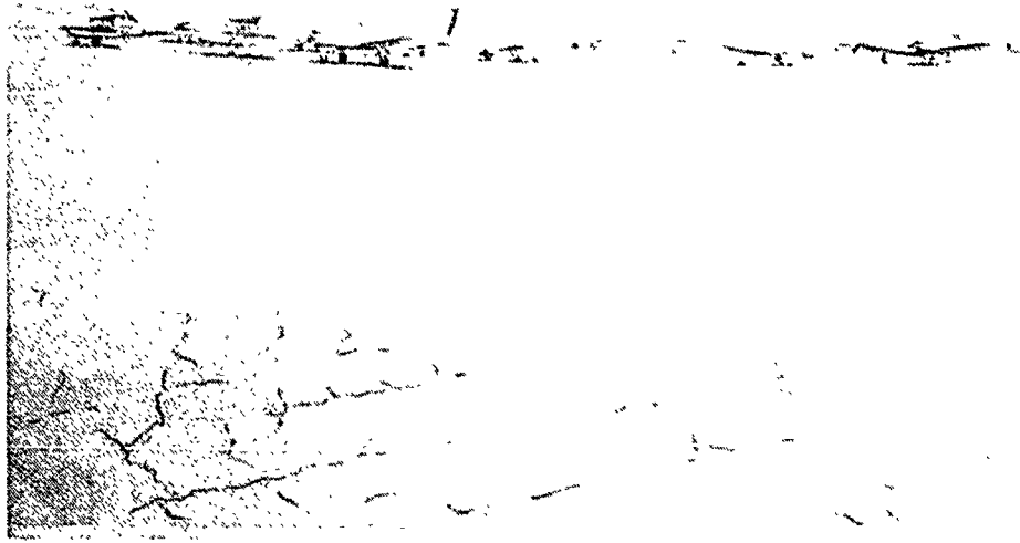
Photo 3 Coal tar emulsion seal coat using heavy sand loading on new asphalt pavement showing crack pattern developing (Florida)
